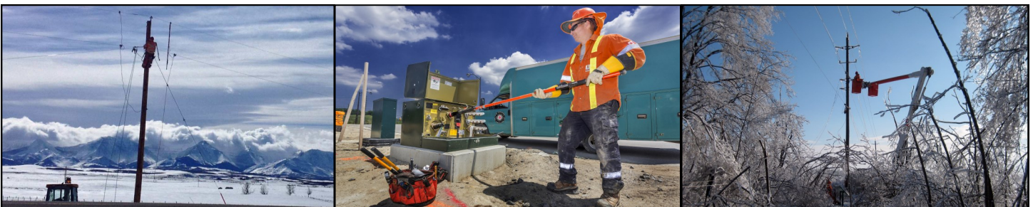
Scope: K-Line Maintenance & Construction Ltd., K-Tek Electro-Services
